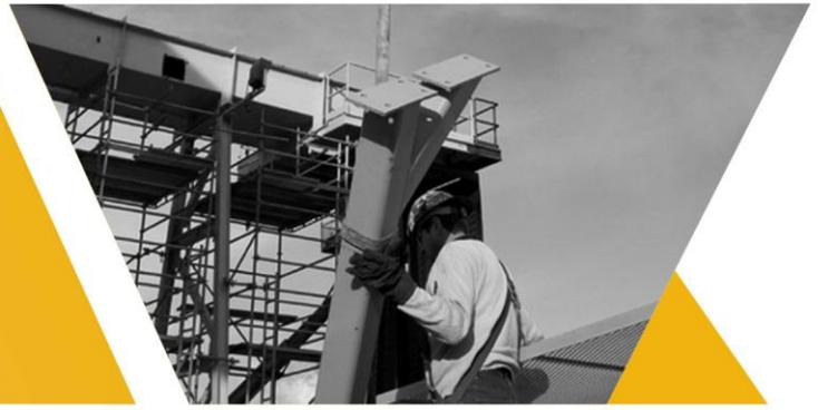
**Description** Riggers assemble and install rigging gear such as cables, ropes, pulleys and winches to lift, lower, move or position machinery, structural steel and other heavy objects.
